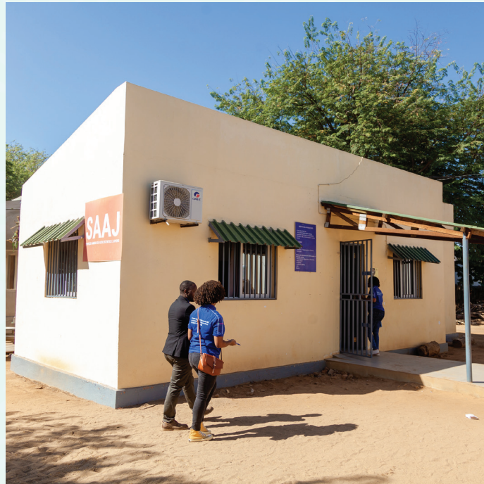
ICRH-M health centre in Changara
